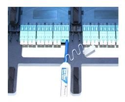
Take out the LC 900um connectors from the RAKE tool and clean them on the lintfree wipes.
