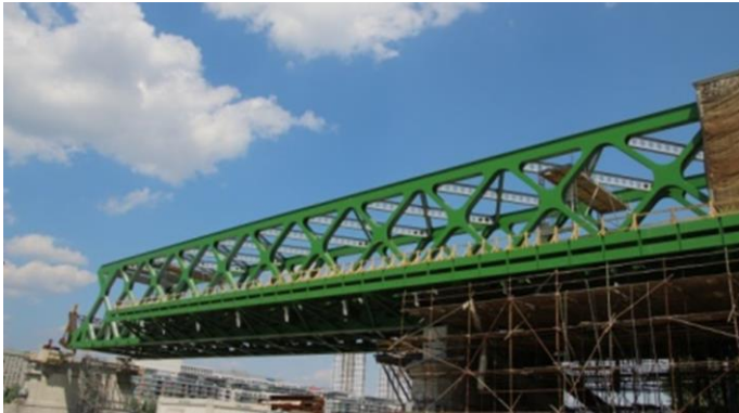
Figure X: Incremental Launching Method
