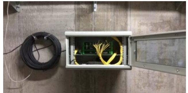
Integrated measurement instruments and optical distribution cable
